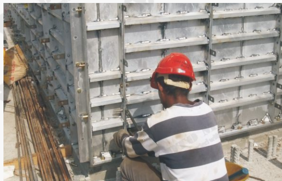
Assembling inner & outer wall panels
