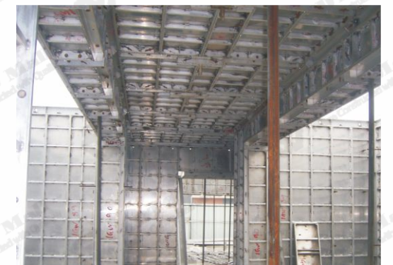
Assembling slab panels
