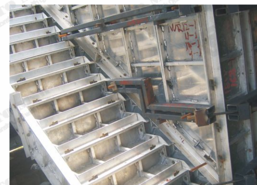
Assembling staircase
