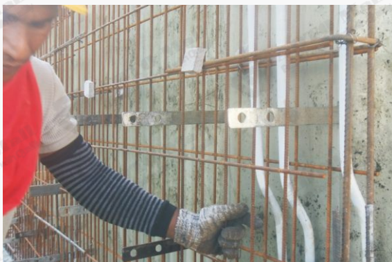
Assembling tie plate
