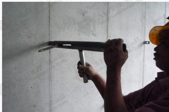
Assembling inner & outer wall panels
