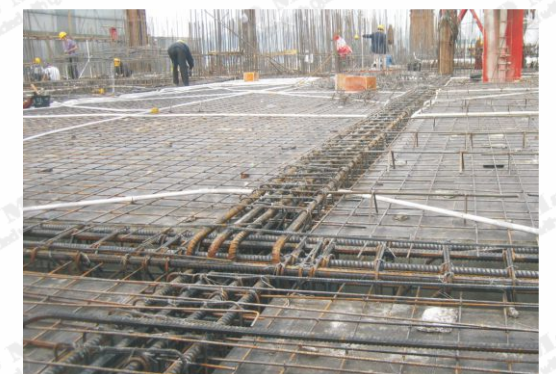
Binding rebars and assembling wire&pipes
