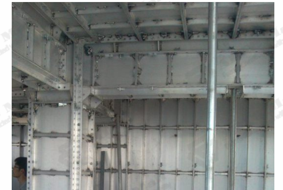
Assembling column
